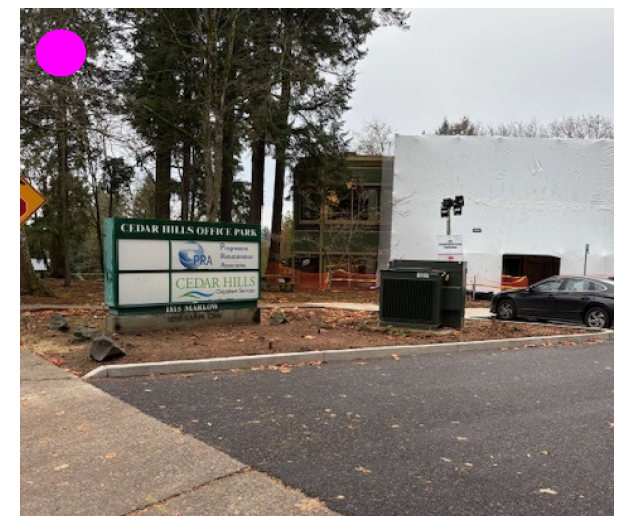
View of building from SW Marlow Ave
